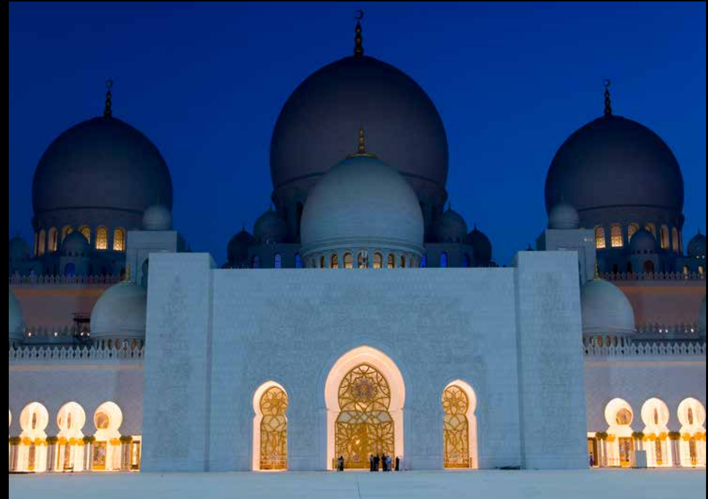
Sheik Zayid Mosque, Abu Dhabi / United Arab Emirates. Architecture: Yusef Abdelki, Syria (design), Halcrow International Partnership, Dubai / United Arab Emirates (execution). Interior design: Spatium Architects, Milan / Italy. Lighting design: Speirs + Major, Edinburgh / Scotland.
