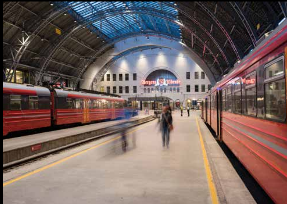
Jernbanestasjon, Bergen / Norway. Lighting design: Ruth Marie Bottenheim. Photography: Johan Elm, Stockholm / Sweden.
